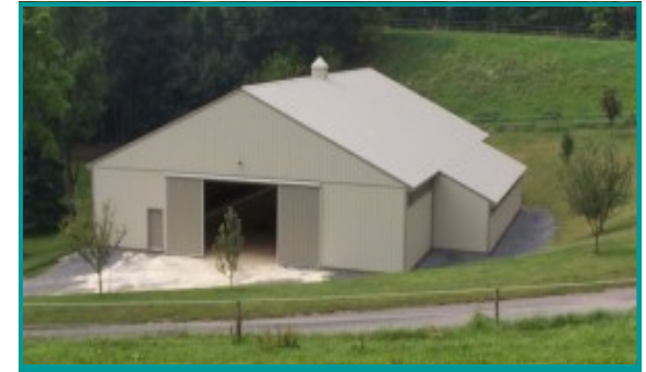
65' X 96' indoor arena with sand/sawdust footing. Dust free and well maintained. Excellent lighting and ventilation for your comfort.
